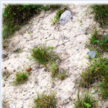
Above: Master plan of the DPFLI illustrated by Hagenbuch Weikal Landscape Architecture. Right: Cracked soil surface at the DPFLI indicating low organic matter and compaction.
