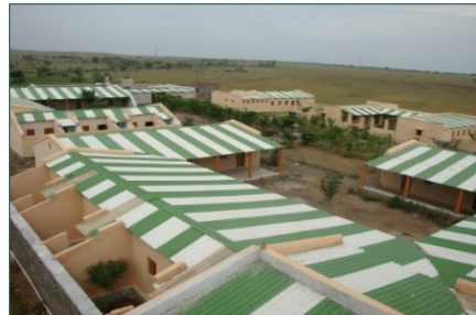
Figure 17-4. Huge infrastructure at Palshi Village, Baramuti.
