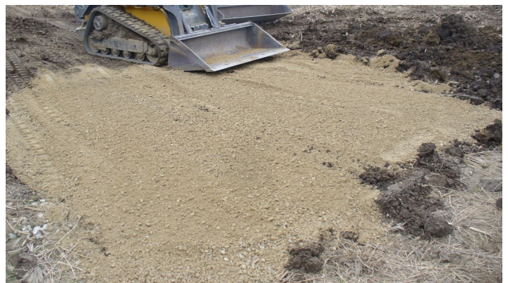
Figure 1- Left: A surface inlet before being replaced by a blind inlet. Right: the finished blind inlet (photo credit: Justin L. McBride)
