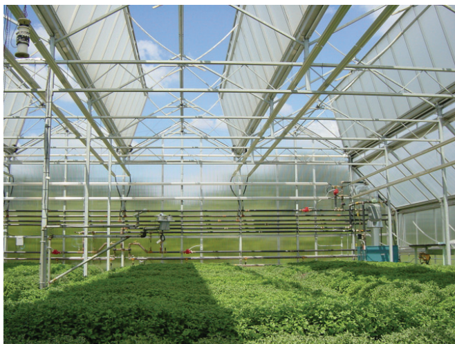
Figure 10. Open-roof greenhouse with a fall chrysanthemum crop. Note the shadow bands on the crop caused by the cover material (double poly) on the greenhouse roof. Photo courtesy of A. J. Both, Rutgers University.
