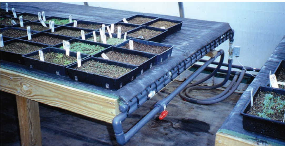
Rubber tubing and PVC pipe are used to supply this flat-top root zone heat mat. PVC pipe can handle up to 130° F water without sagging.
