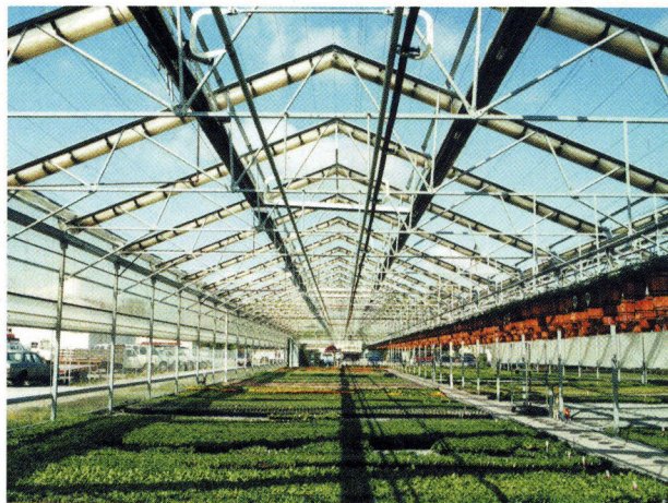
A row of infrared heating units is suspended on each side of this retractable roof house. Bedding plants are growing on the floor and hanging baskets line the side aisles.
