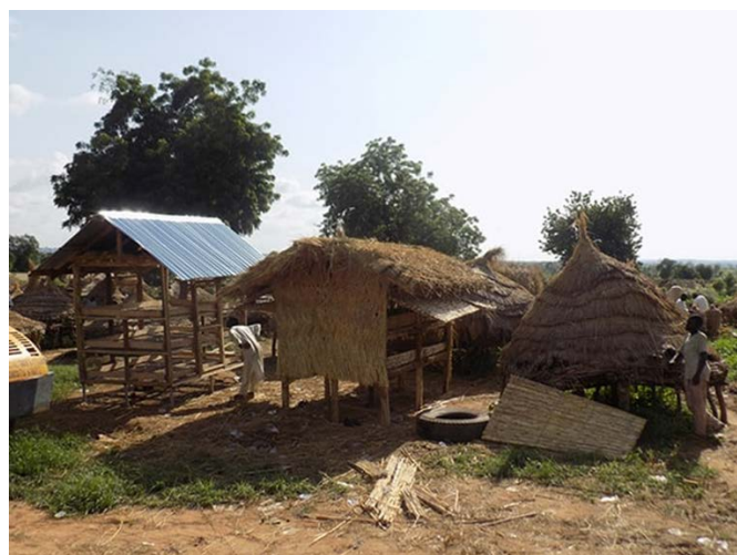
The traditional “ Rudu ” used in storing onions alongside the improved structure that allows for better aeration.
