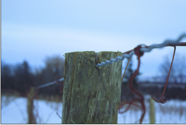
Fig. 33. The groove in the top of this vineyard post provides excellent support of the trellis wire and still allows post pounding without damage to the wire.
