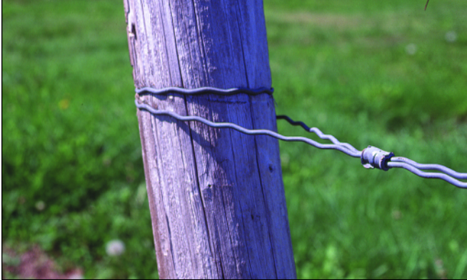
Fig. 35. A high-carbon trellis wire that has been attached to an end post by wrapping the wire around the post and then attaching the wire to itself with a soft-metal crimp.
