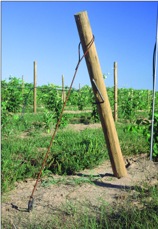
Fig. 29. This end post was set with a 30-degree angle from vertical. Reinforcement rod connects the post to the anchor and an L-shaped crank is being used to tighten the one wire attached to this post.
