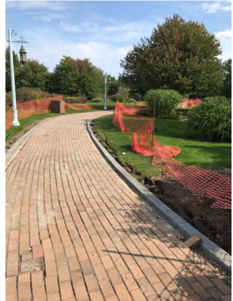
The walkway under construction
