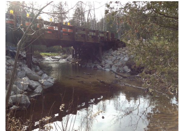
Photo 4-6: The bridge that replaced the road culvert river crossing in Photo 4-5 protects the river from sediment and reconnects the fishery to the Great Lakes.
