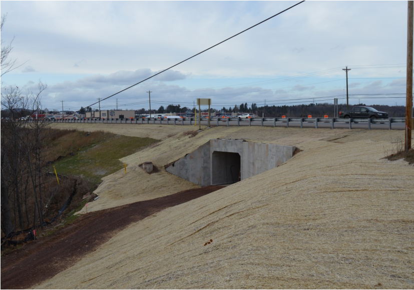
Newly constructed underpass below the corridor
