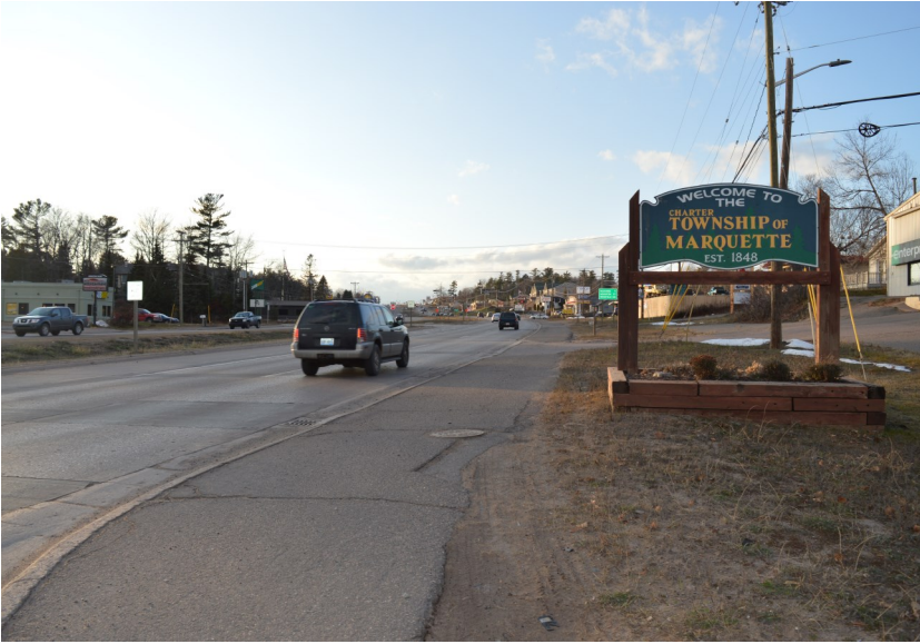
Graded shoulder used by pedestrians and bikers along corridor
