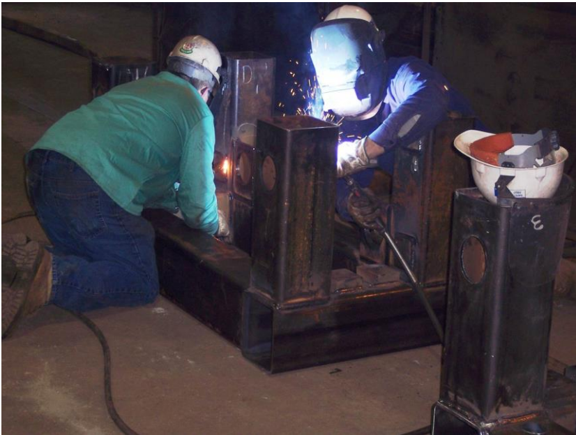
Workers kneeling during fabrication
