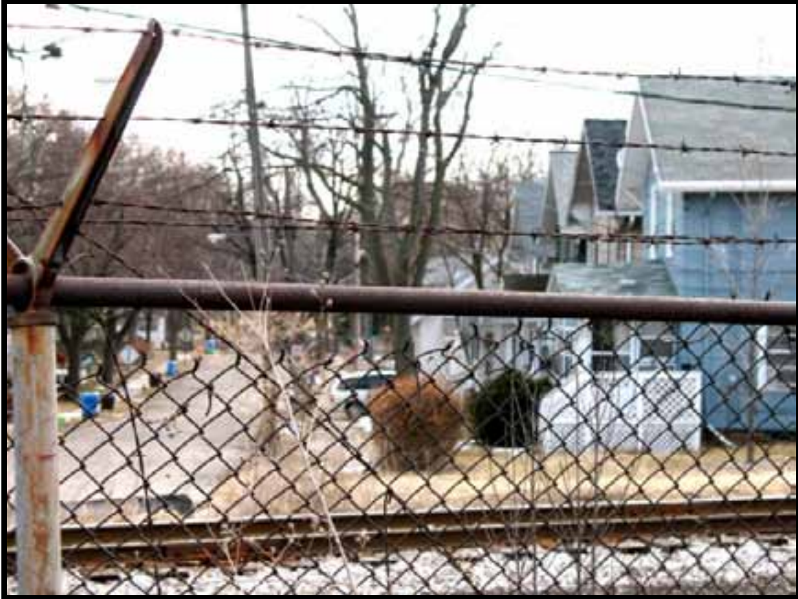
Figure 2.5 Residential homes directly adjacent to the John Bean Building with no buffer
