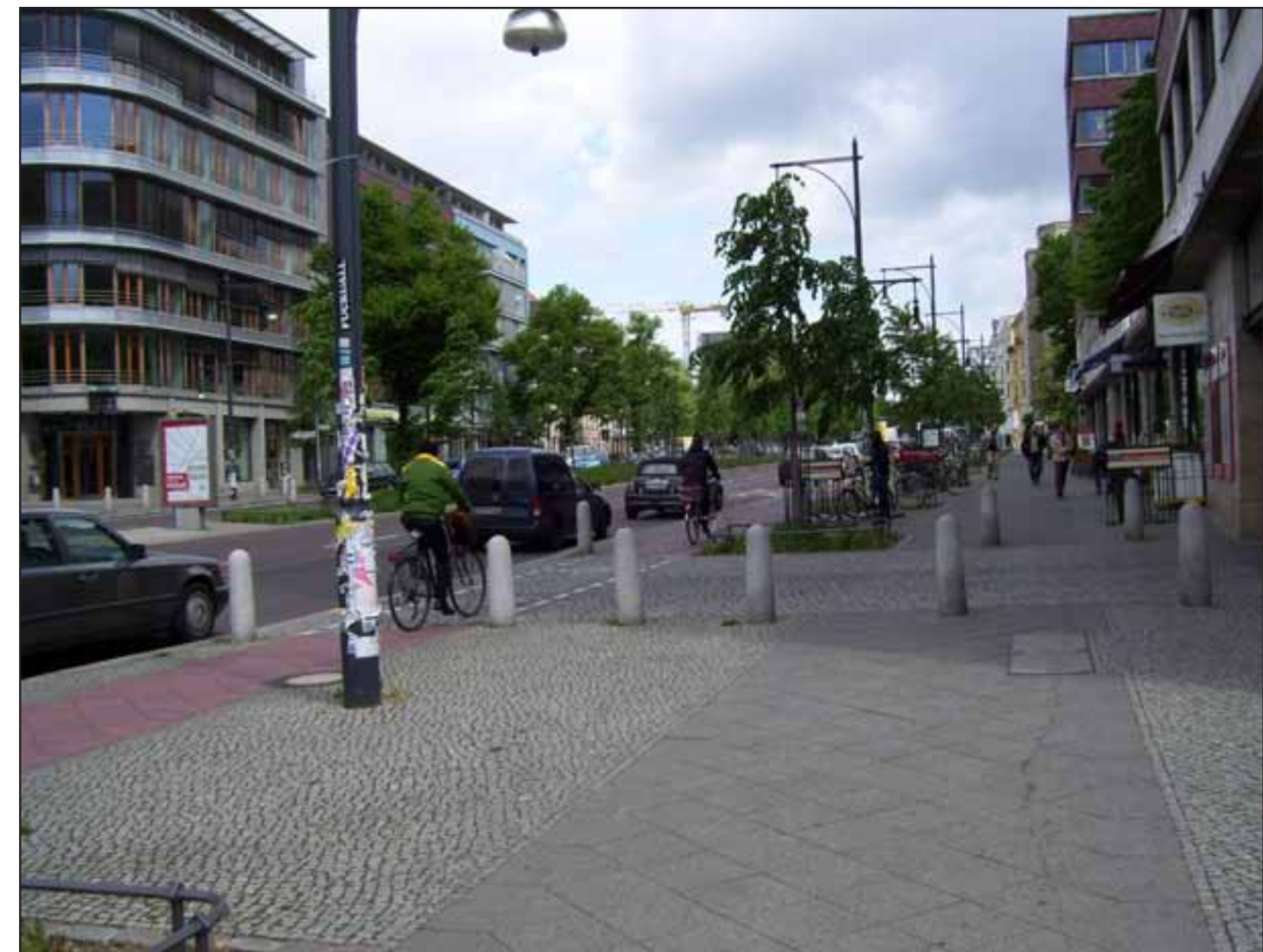
Non-Street Grade Bike Lanes, Germany
