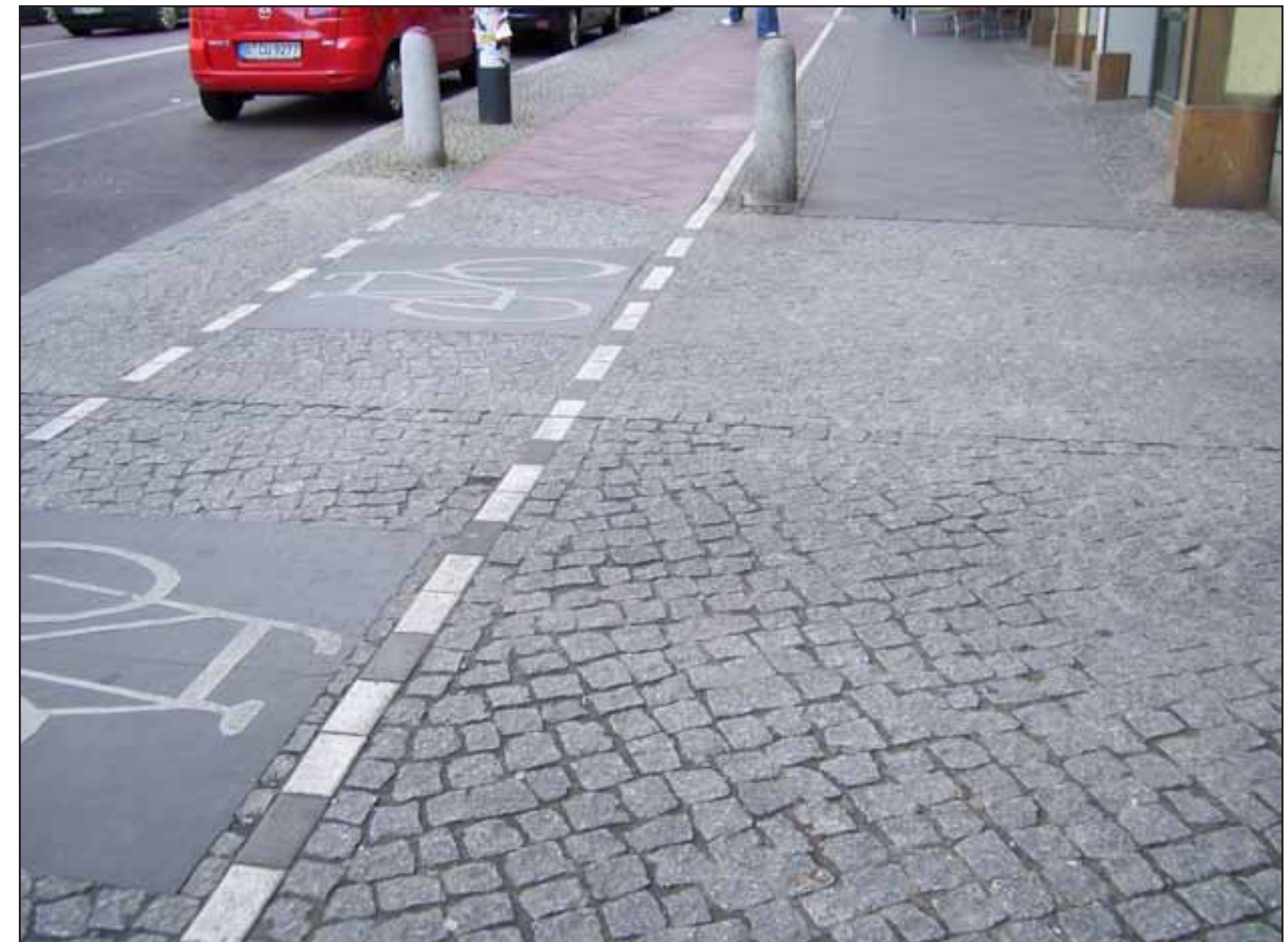
Non-Street Grade Bike Lanes, Germany
