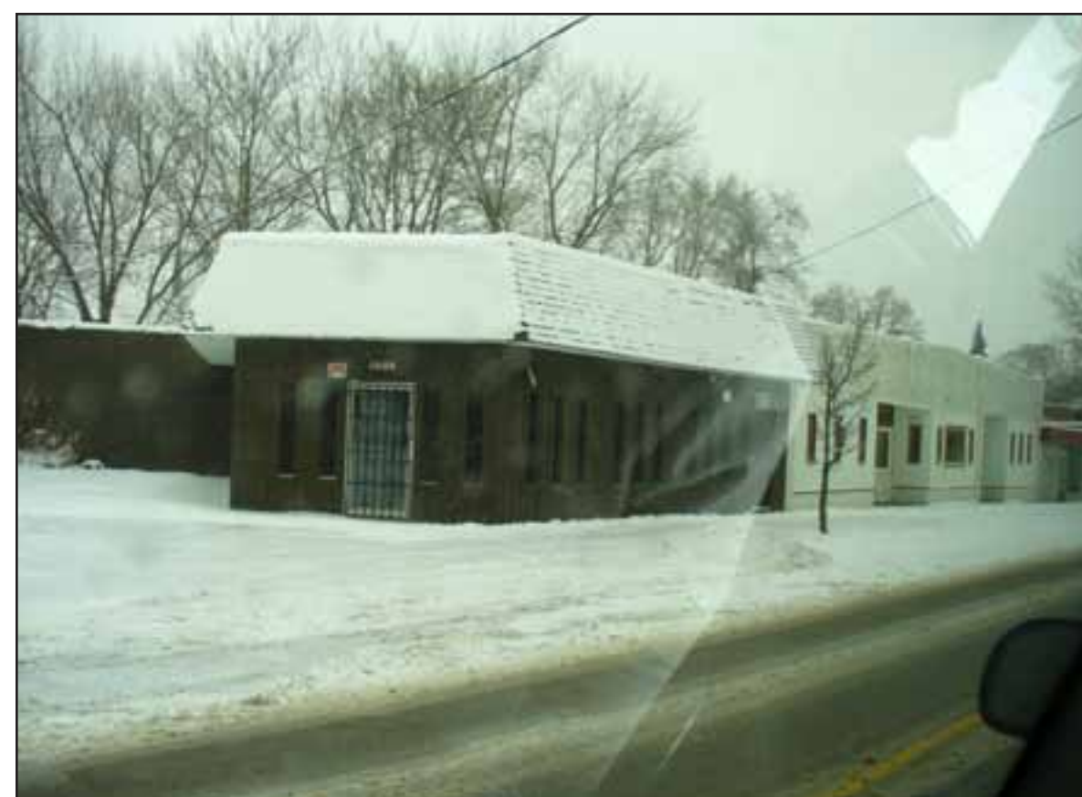
Abandoned Key Shop
