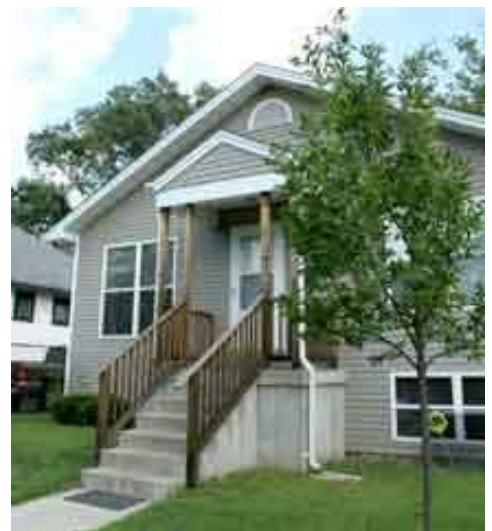
A rehabilitated home in St. Louis. Source: www.beyondhousing.org
