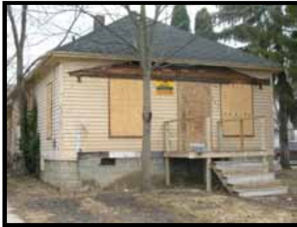
A vacant structure in the study area
