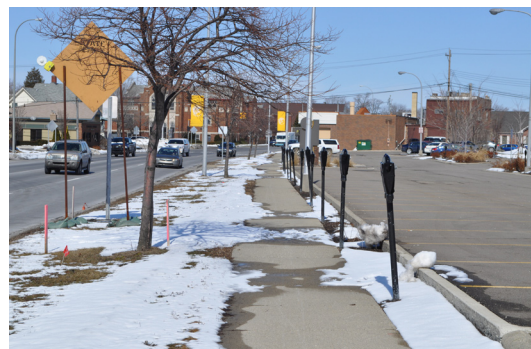
Figure 3.11 Narrow Sidewalk and excessive block length.
