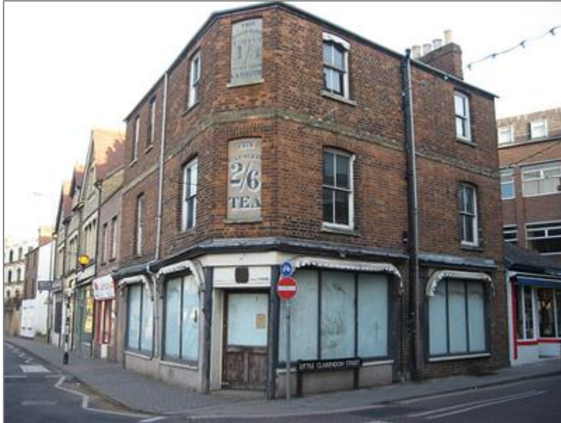
Figure 4.2.2.1 – ‘Fair’ Structure Example
