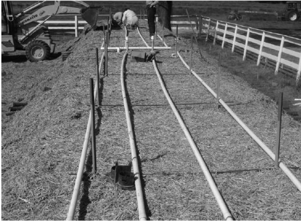
Figure 1: Filter mound under construction.
