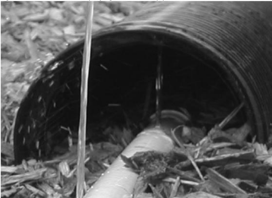
Figure 2: Distribution line spraying under round pipe.
