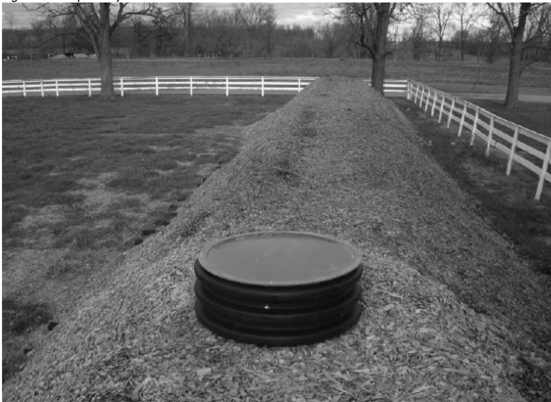
Figure 3: Completed filter mound.
