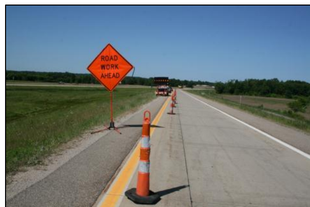
Safety equipment necessary for highway sites. Photo courtesy of Dennis Pennington.
