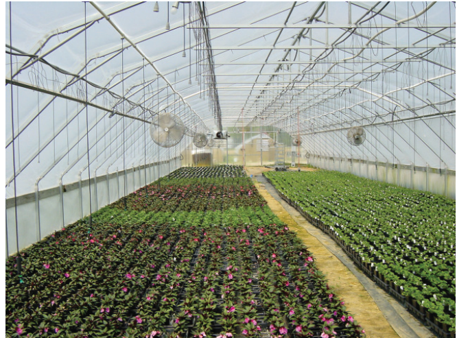
Figure 9. Horizontal airflow fans (HAFs) installed in a greenhouse to increase the uniformity of growing conditions. Photo courtesy of A. J. Both, Rutgers University.
