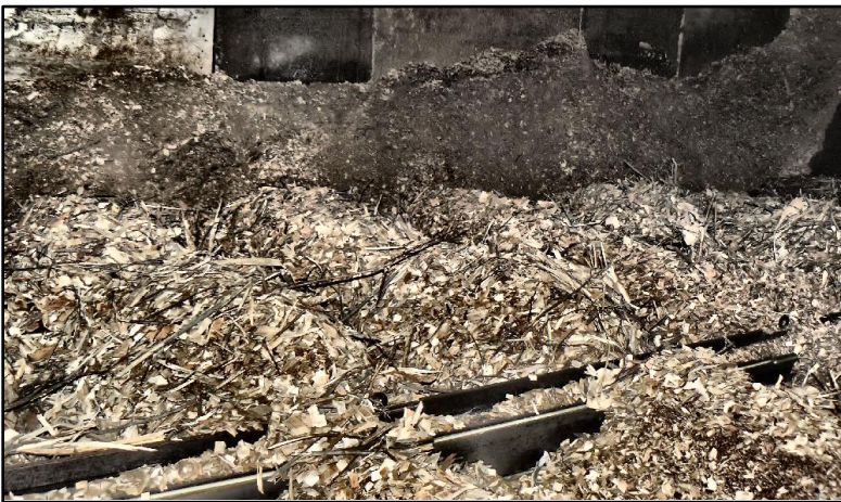
Above: wood chip storage bin with walking floors.
